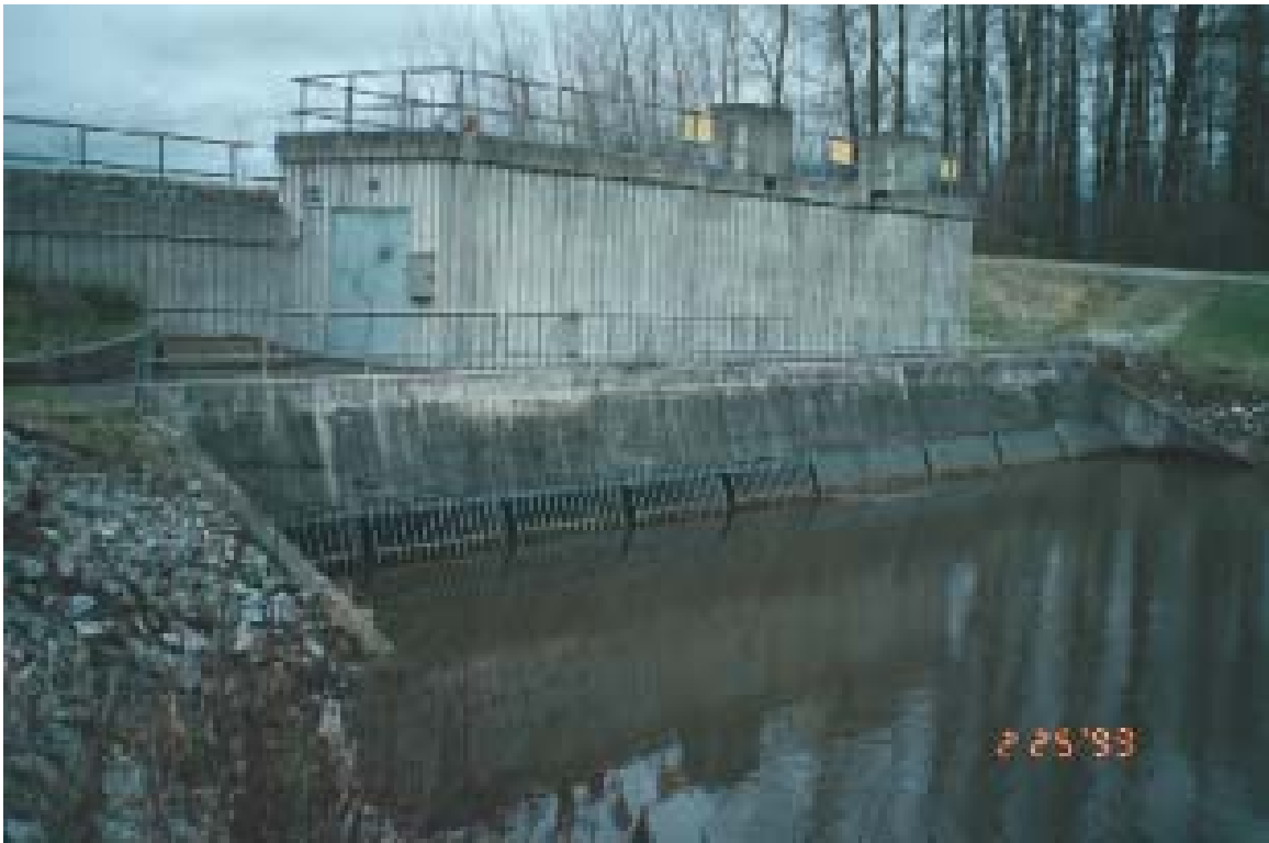
Photo 3: Katie Slough station: pump intakes (R), flood box entrance (L).
