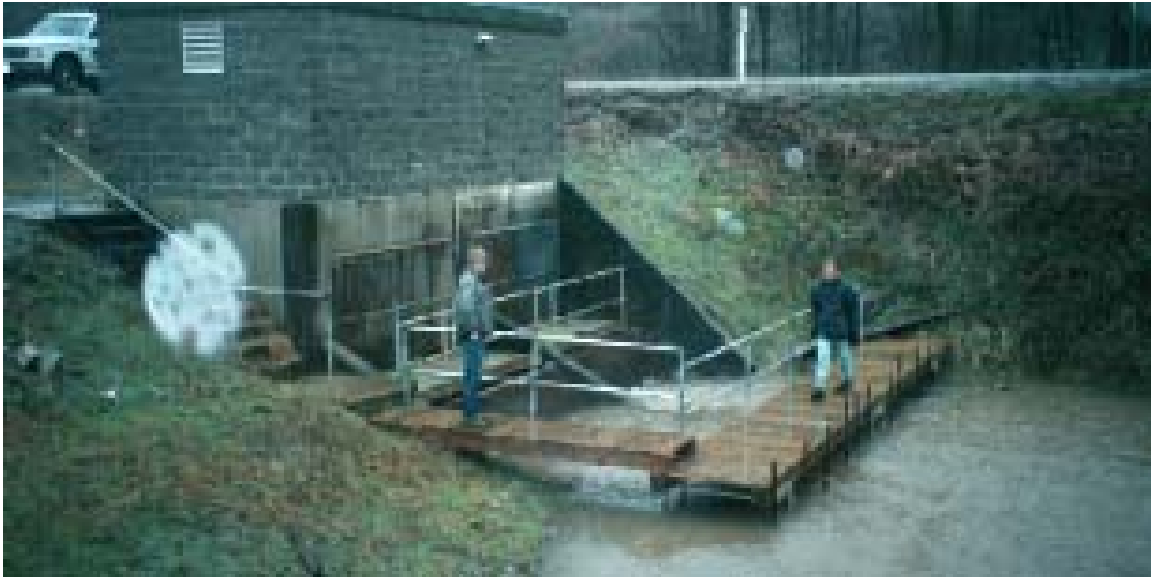
Photo 19: Silverdale station (Chester Creek): walkway to facilitate fish salvage during freshet.
