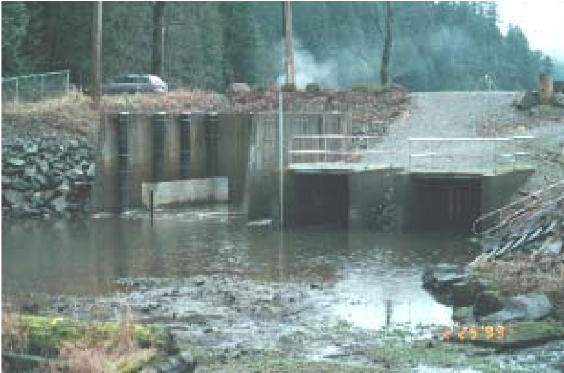
Photo 11: Miami Creek station: flood box entrance (R), future pump house sump (L)
