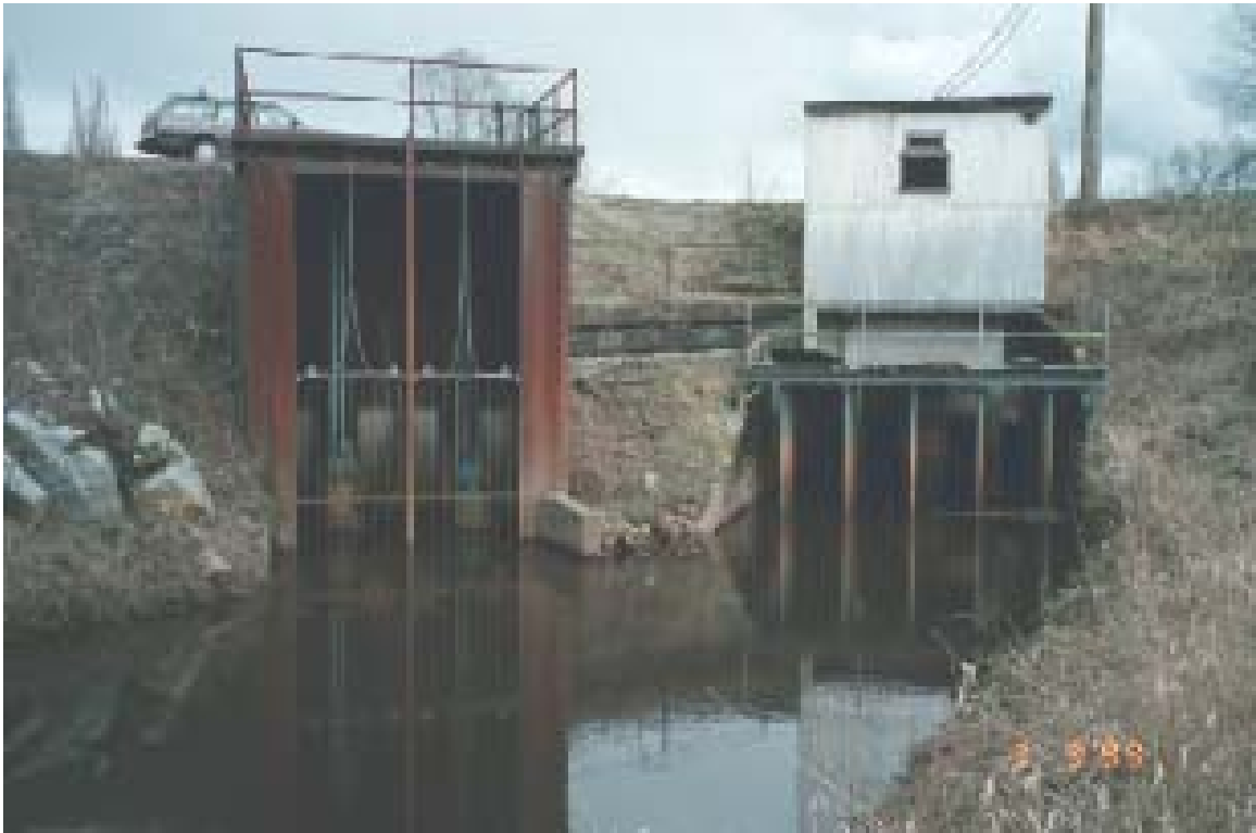
Photo 17: Nathan Slough station: older station (R), new station (L) with submersible pumps.
