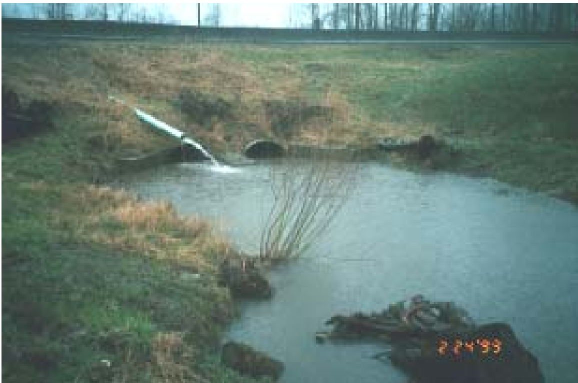
Photo 22: Lane Creek station: culverts lead to pump station behind embankment.
