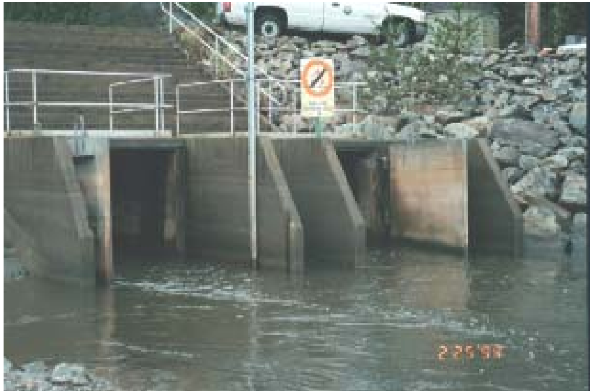
Photo 11: Miami Creek station: flood box entrance (R), future pump house sump (L)
