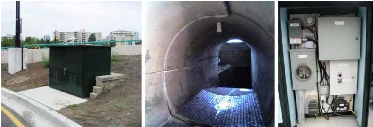
Heather CSO kiosk, sampling tube installation in Balaclava CSO and kiosk electronics
