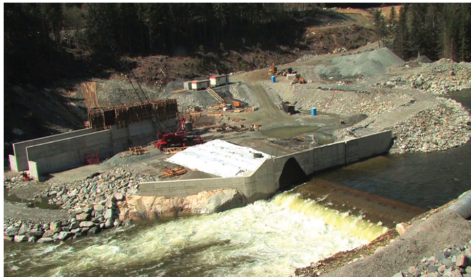
Ashlu River diversion under construction
