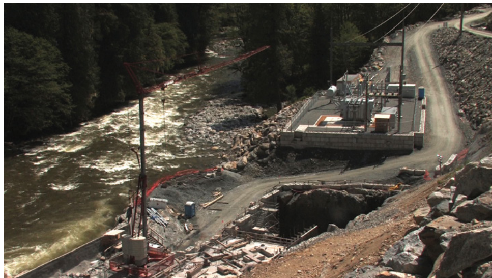
Ashlu River powerhouse under construction
