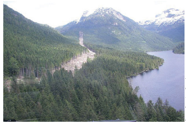
Transmission line near Freda Lake in the Sunshine Coast
