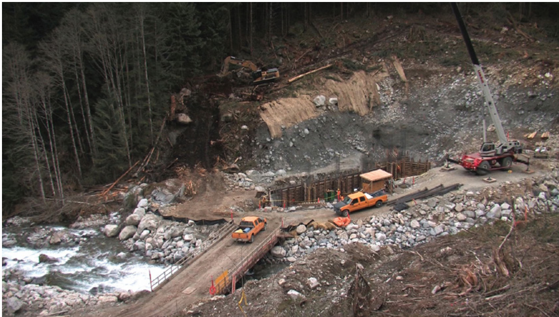
River diversion construction at Tipella Creek near Harrison Lake
