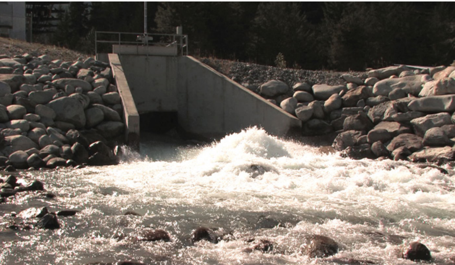
Water leaving the powerhouse on Rutherford Creek
