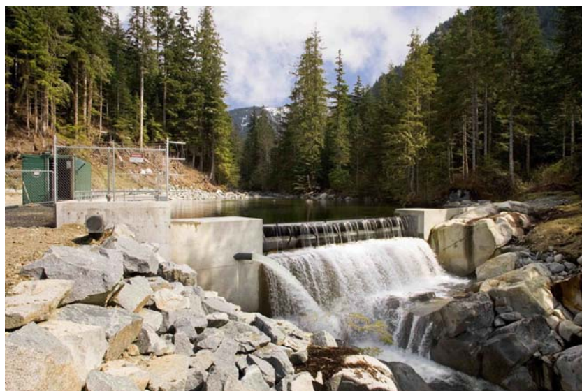
Figure 5: Weir, intake and headpond at Furry Creek.
