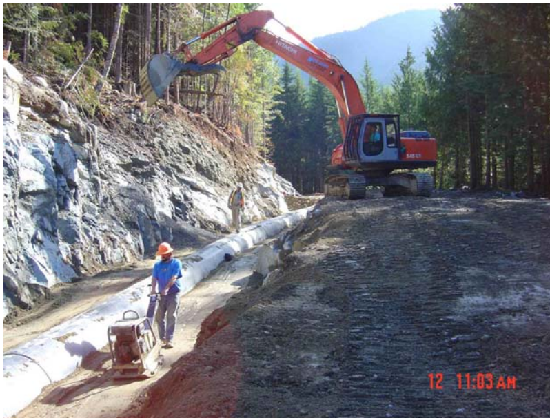
Figure 7: Construction of penstock at Furry Creek.
